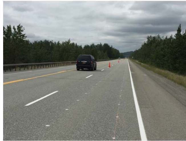
2-Lane Road, Passing Area, Alaska
